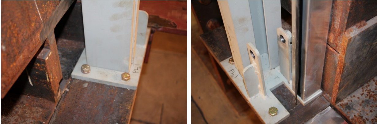
Figure 17. Baseplate Connection
