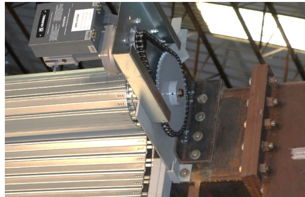
Figure 16. Roller Shutter Mounting
